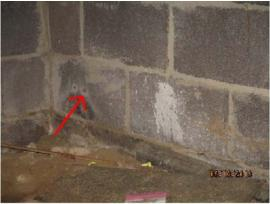
Vertical crack noted on foundation wall in rear crawl space. No deflection. The crack appears to be static and does not threaten the integrity of the structure.
